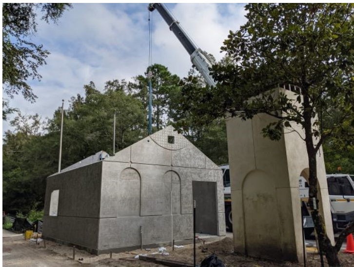
LEFT: The four pre-fabricated concrete walls of the new ranger station were installed on Thursday, September 2. RIGHT and BELOW: Blueprints of the completed ranger station and its interior.
